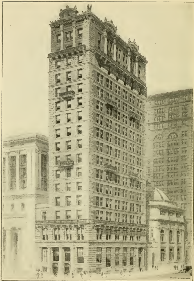
AMERICAN EXCHANGE NATIONAL BANK. 128 Broadway, northeast corner Cedar St.
